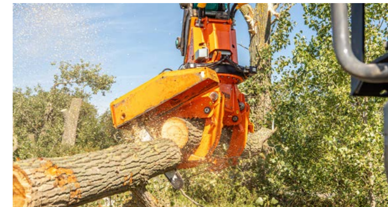
Rapid chopping and piling.
