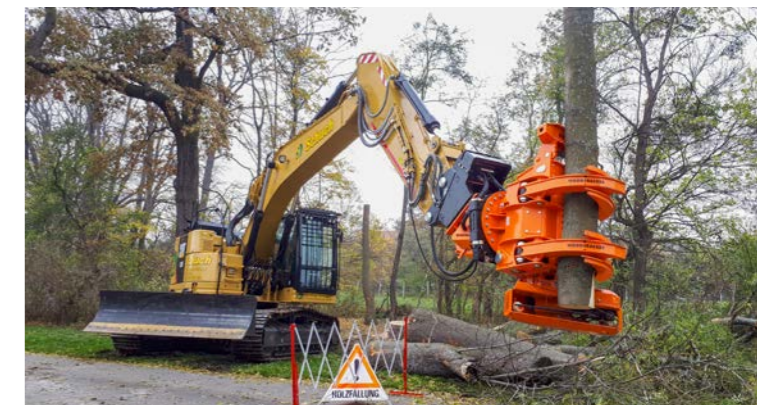
Maintenance work along traffic roads and routes.
